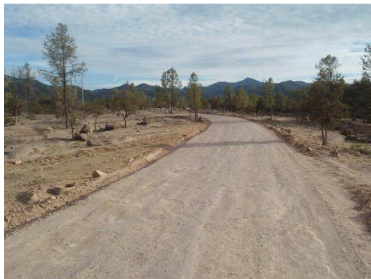
Figure 1: View of Km. 10 + 000 Back View
