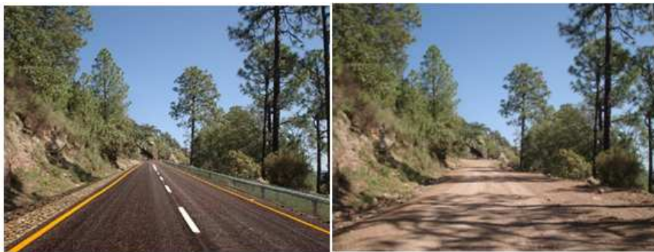
Figure 29: Example of the Road with a Gutter of Regional Materials and Flexible Defense with Treated Wood, Road of Cerocauí. Chihuahua Source: Self -Made
